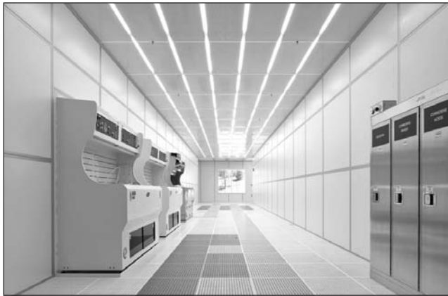
One of the new cleanroom bays in the expanded LNF.
